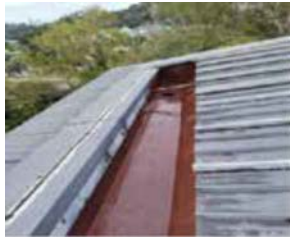
Badminton court gutter repair
