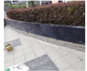
Damaged drain repair
