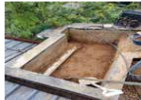
Plant box repair
