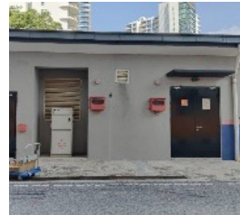
Painting mechanical room
