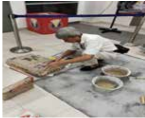
Repair of damaged tiles
