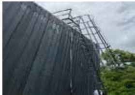
Monkey Ladder Installation
